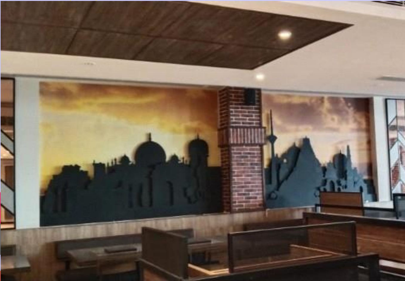
VINYL PASTED ON BACKGROUND WITH 3 LAYERS LASER CUT MONUMENT
